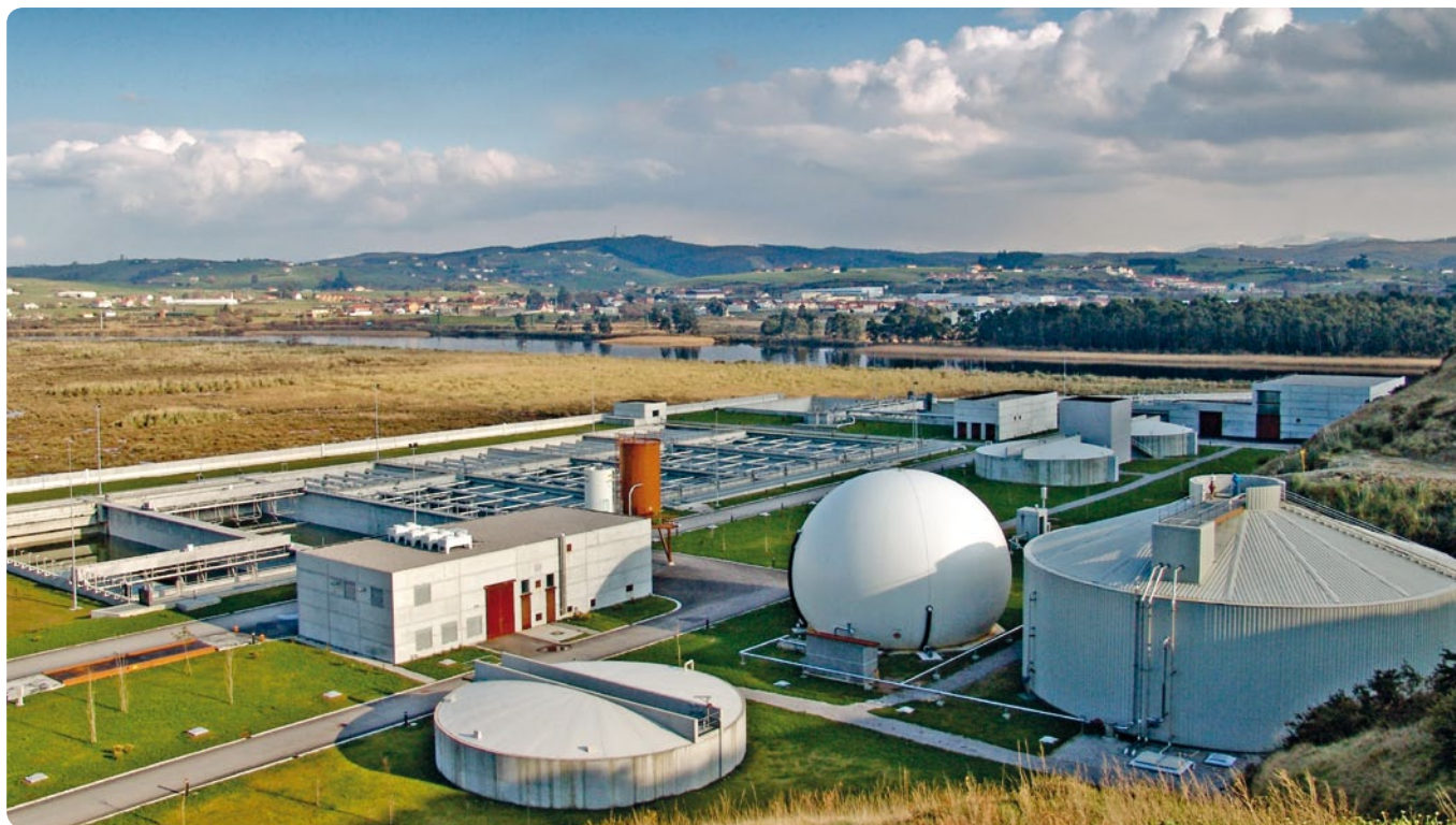
WASTEWATER TREATMENT PLANT, SUANCES, CANTABRIA.
