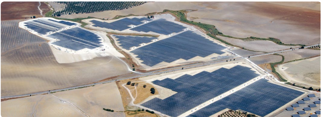
PHOTOVOLTAIC SOLAR FARM, ESPEJO, CÓRDOBA.
