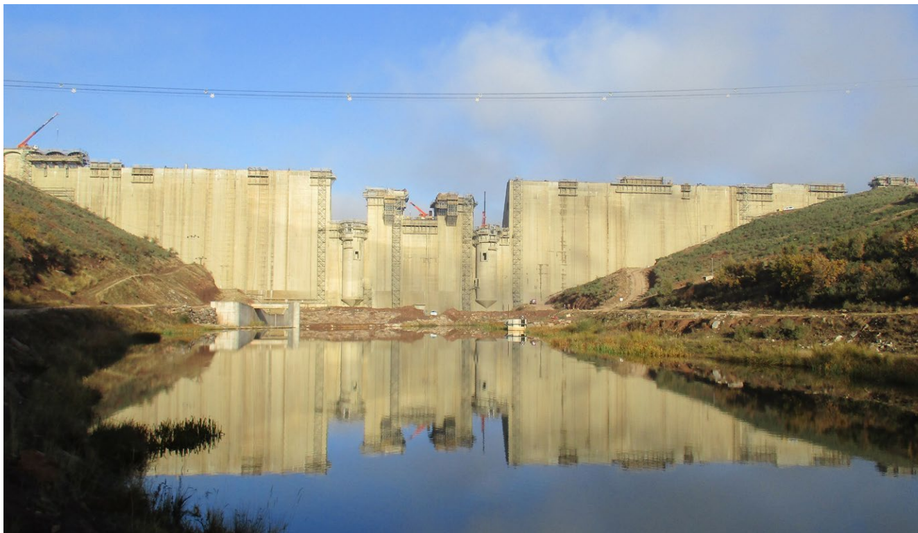
Castrovido Dam, Burgos (Spain)
