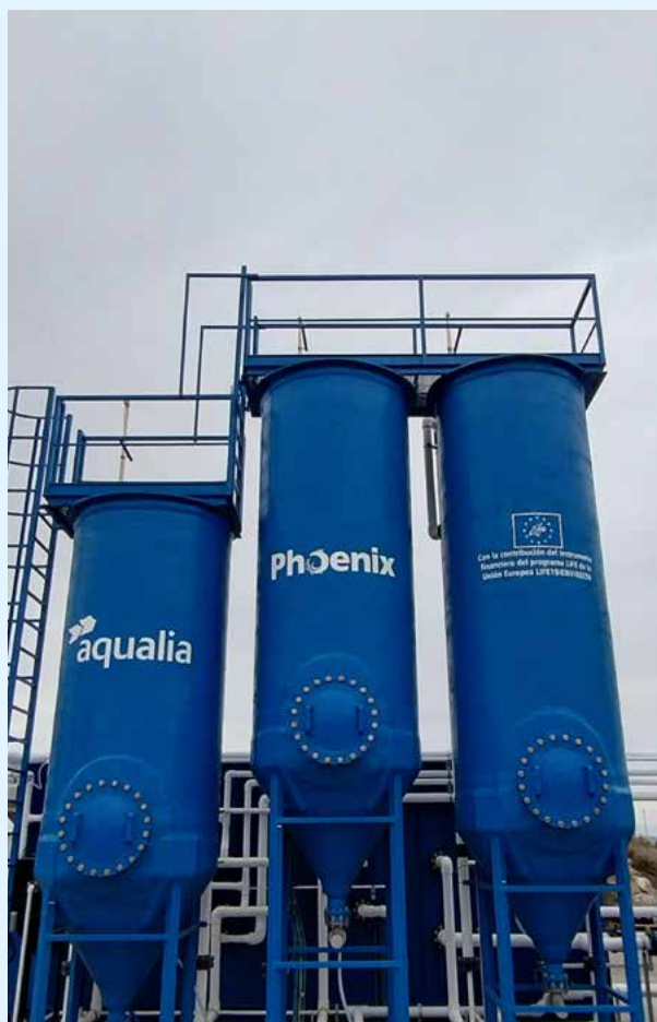
From right to left, skid of continuous and semi-continuous wash filters; and disinfection container with UV, O 3 , and H 2 O 2 .
