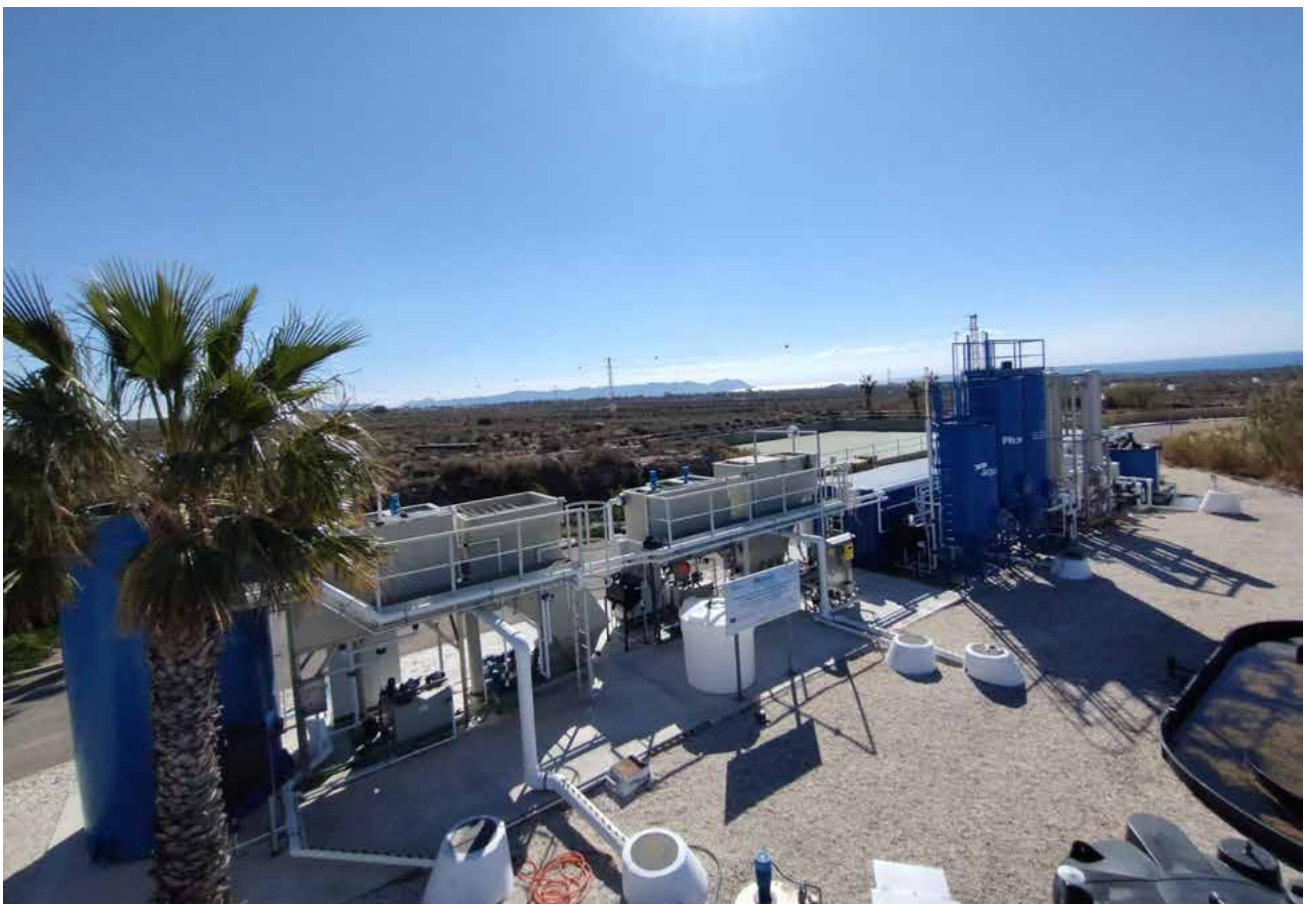
Aerial view of REUSA Hub.
