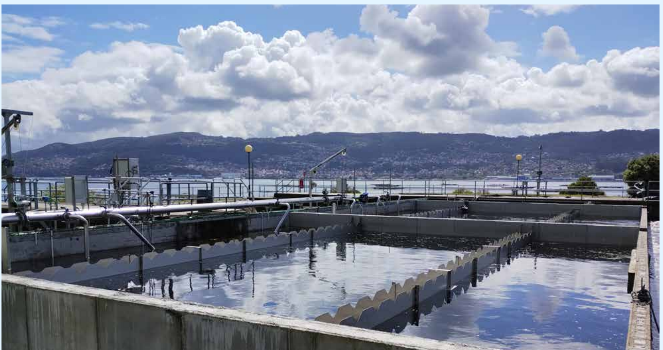
Granular reactors of the LIFE RESEAU project at the Moaña WWTP.
