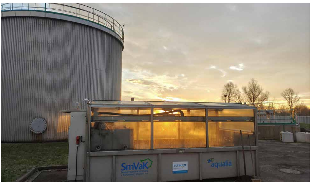
Sludge drying using a solar system.
